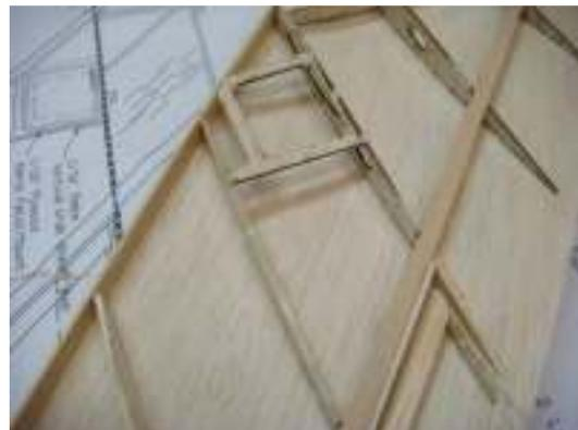
Glue the 1/16" plywood servo hatch mount in place. At the L.E. make sure
